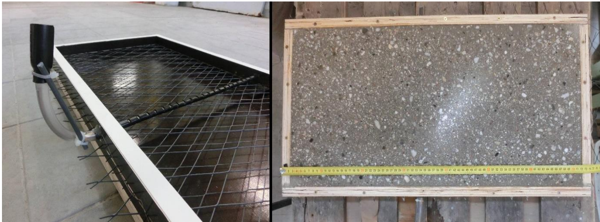
Figure 3: Installed liquid junction (left), concrete base plate (right)
